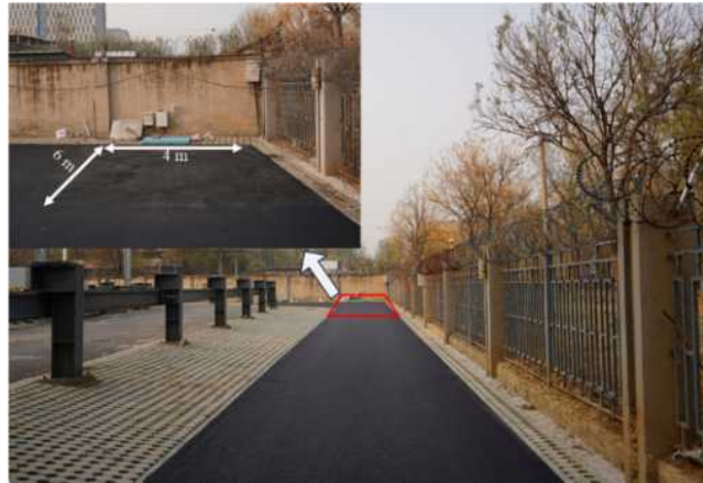
Fig. 1 A trial section of asphalt pavement for oxygen measurement and monitoring
